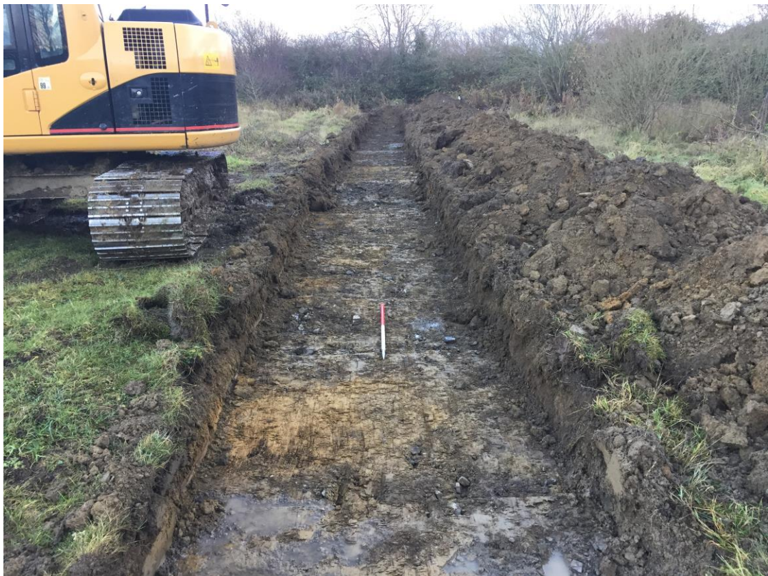
Plate 40: Field 10 Trench 1, looking south east
