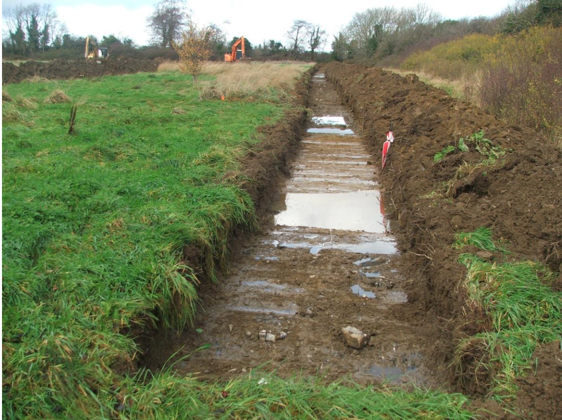
Plate 17: Field 6 Trench 1, looking north west
